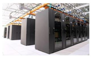
HPC hardware is housed in liquid-cooled enclosures in UW IT's 6,000 sqft data center which includes highly redundant infrastructure for power, cooling, and security. Hardware is interconnected utilizing Mellanox InfiniBand and high-speed internet. Beartooth's condo-style heterogeneous environment hosts specialty nodes to address a wide array of compute requirements including mass memory (4TB RAM) nodes, and a variety of GPU nodes.
